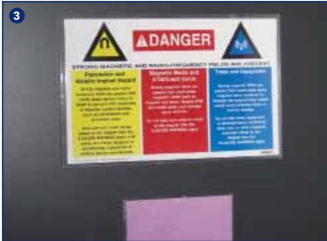
(3, 4) Signs around the entrance to the magnet room. Typically, MRI rooms have signs to warn people entering to be careful, since the magnet is always on. This door is a typical style door that leads into the magnet room. For most MRI scanners, the 5-G line is inside the door, so tools and equipment can be safely brought just to the area outside the door.
