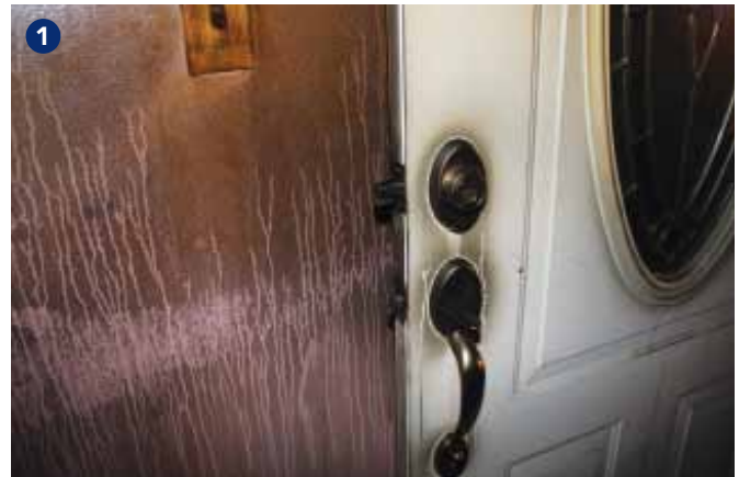
(1) Looking up the latch side of the door slab can help you determine if the door was unlocked or open on arrival and, if the lock was secured, how many locks were engaged. (Photo by author.)
